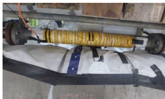
Final laminate being post cured with Heat Tapes
